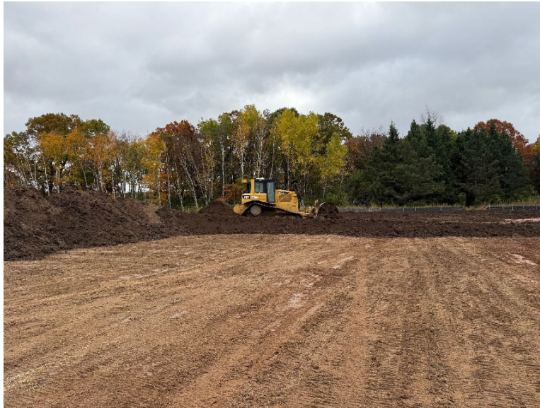
Facing south at MP 0.65, Otis continuing topsoil restoration
