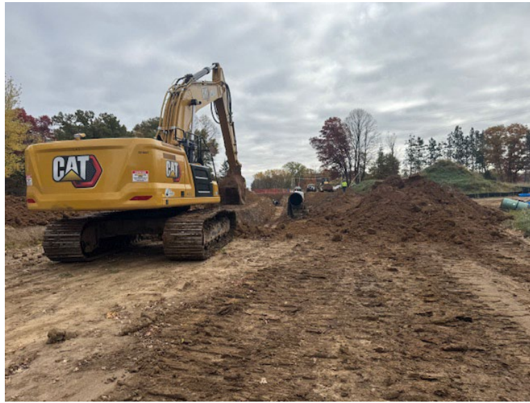
Facing east near MP 2.36, ditching was completed
