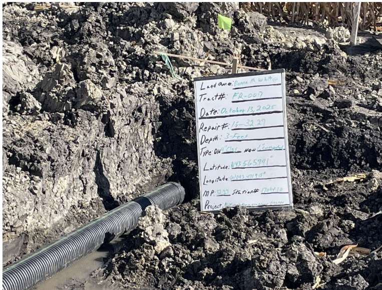
Facing east at MP 32.27, repaired drain tile
