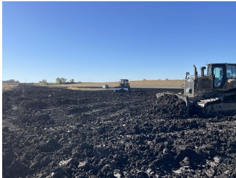
Facing southwest at MP 32.61, K&K restoring topsoil
