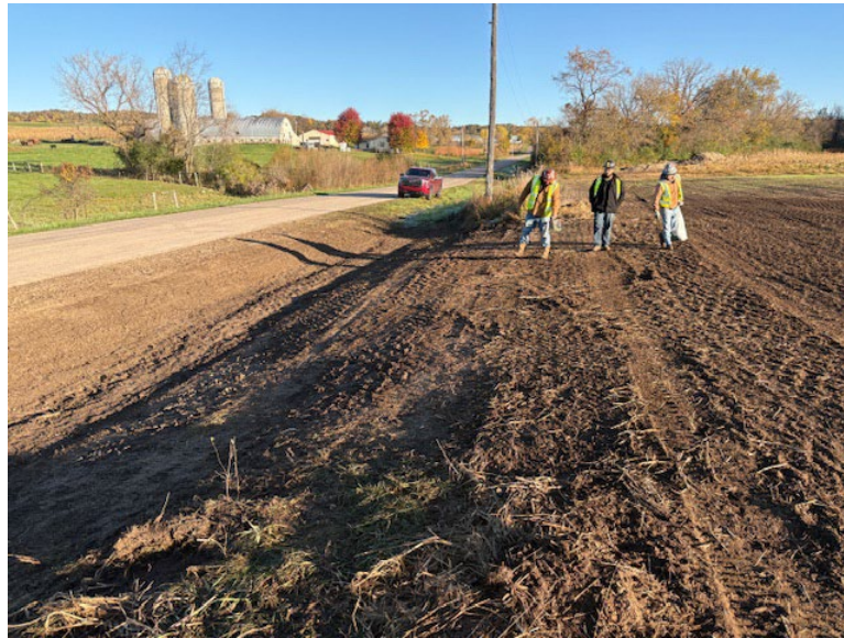
Facing north near MP 3.5, K&K seeding roadside ditch
