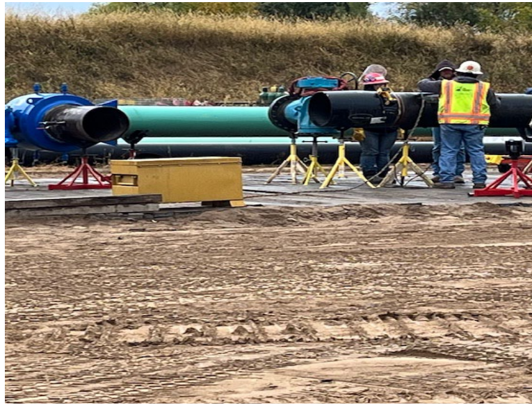
Facing east near MP 1.0, welding pipe fabrication
