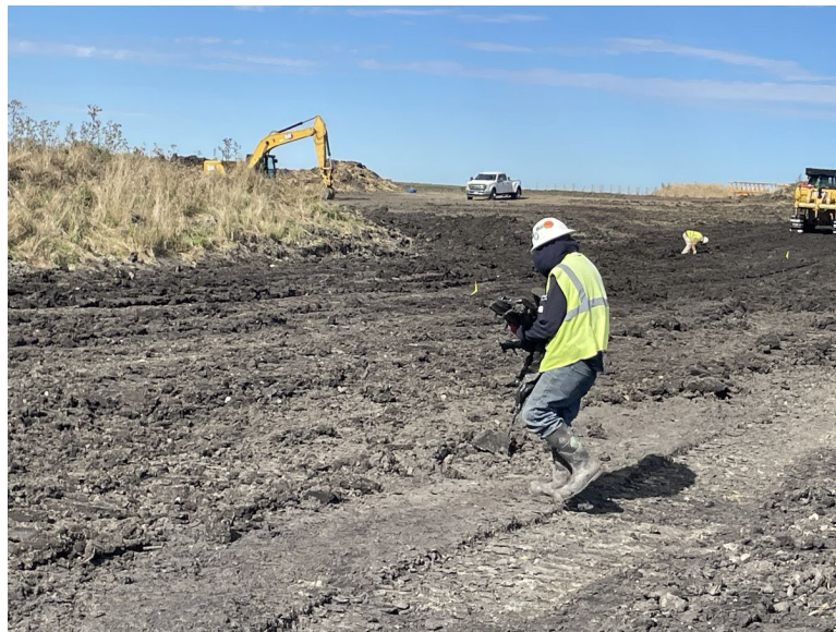
Facing northwest at MP 32.93, K&K removing construction debris (broken mat) from temporary workspace
