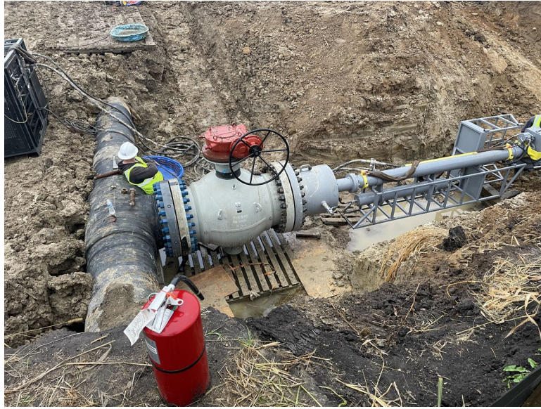
Facing north at MP 34.2, TVT performing D-line hot tap north of 165th Street
