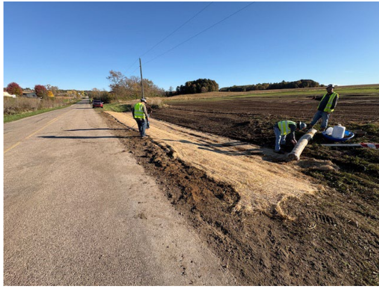
Facing east near MP 3.5, K&K installing ECBs
