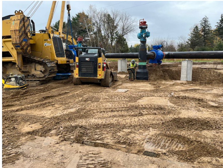
Facing west near MP 3.42, backfill and pier installation completed
