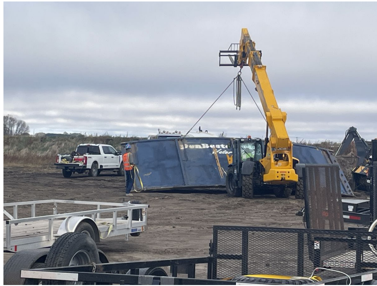
Facing northwest at MP 34.2, Kodiak disassembled lake tank for removal
