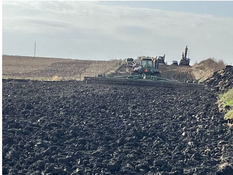
Facing south at MP 32.85, TVT decompacting subsoil north of 140th Street
