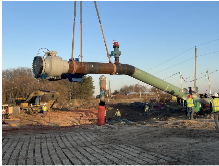
Facing west at MP 34.2, K&K lowering-in tie-over fabrication for the tie-in north of 165th Street
