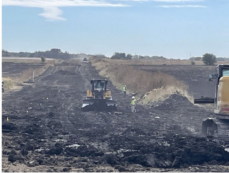
Facing south at MP 32.92, K&K grading subsoil south of 154th Street
