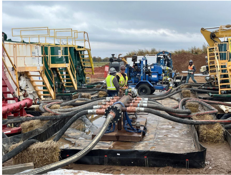
Facing west at MP 0.1, Otis completing the hydrostatic test
