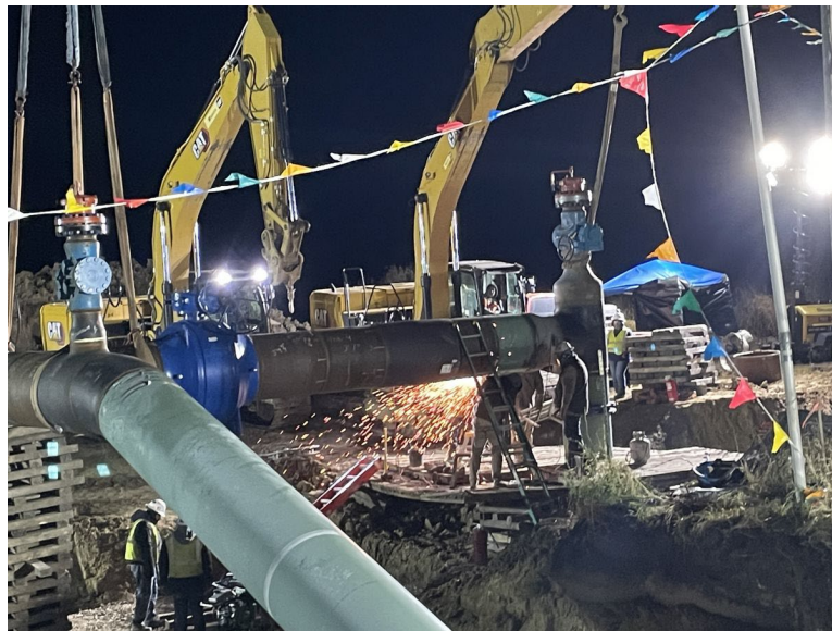
Facing northeast at MP 34.2, K&K grinding a tie-over weld north of 165th Street
