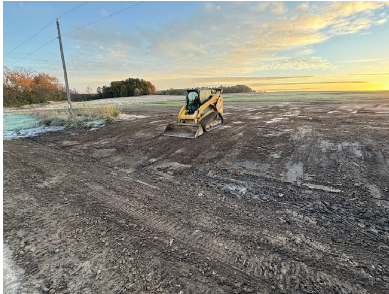
Facing east near MP 3.5, K&K restoring topsoil
