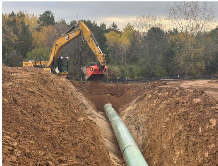
Facing east near MP 1.34, backfill ongoing
