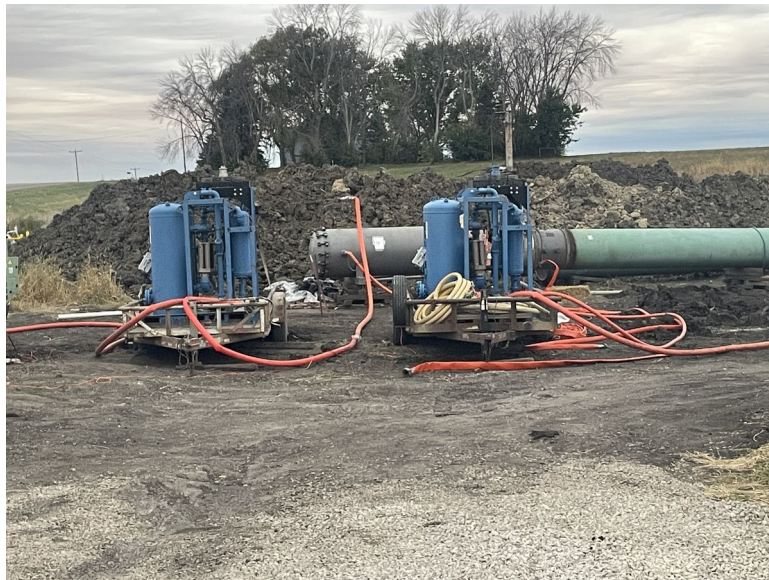
Facing west at MP 31.2, dryers utilized to dry E-line
