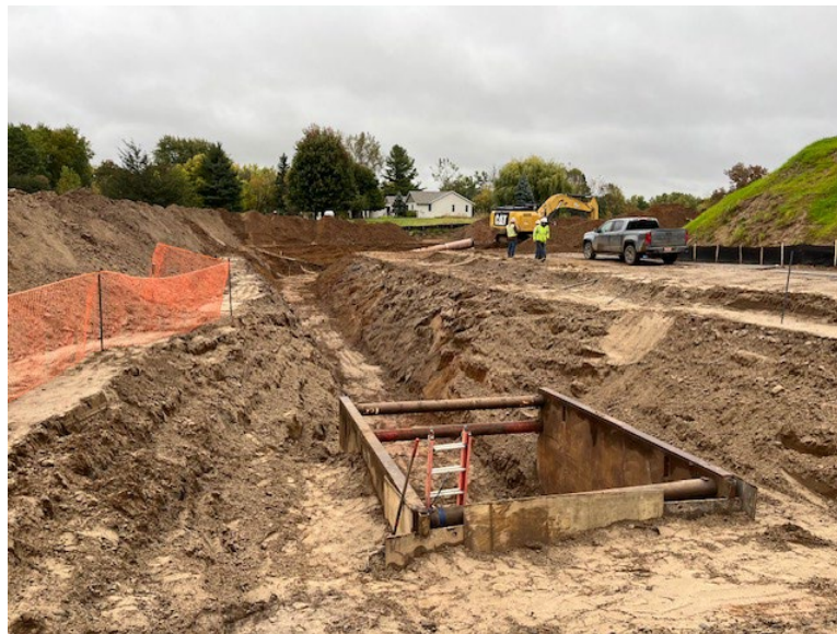
Facing north near MP 1.0, ditching completed for tie-in section
