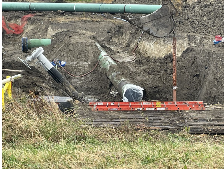
Facing north at MP 31.2, valve setting removal north of County Road 9/135th Street
