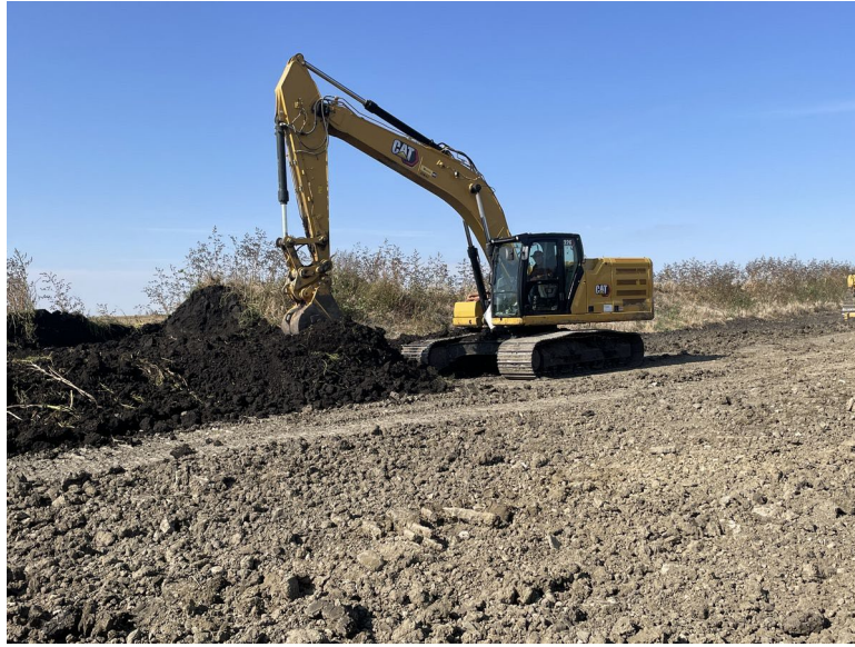
Facing northwest at MP 32.6, K&K utilizing track hoe to pull topsoil
