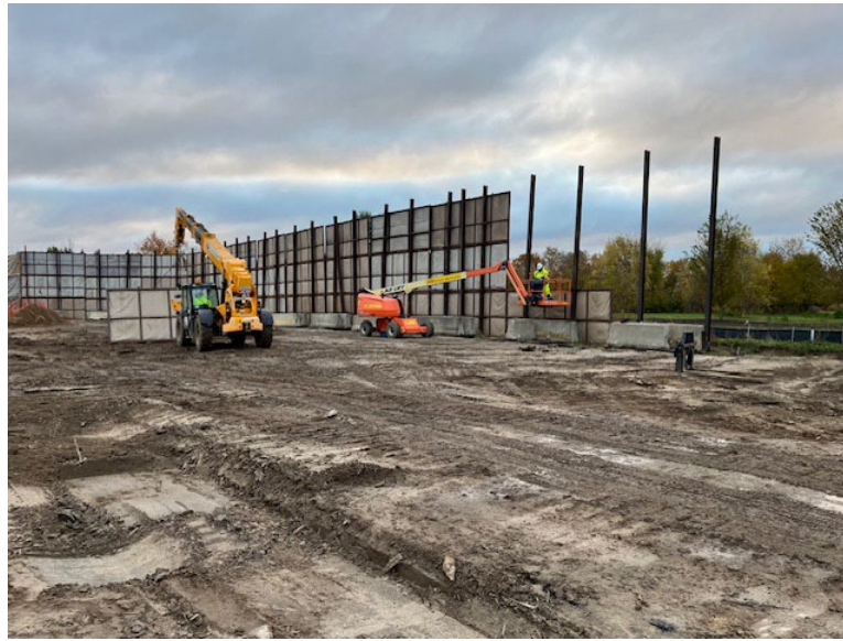
Facing east sound wall removal ongoing for HDD P4-5
