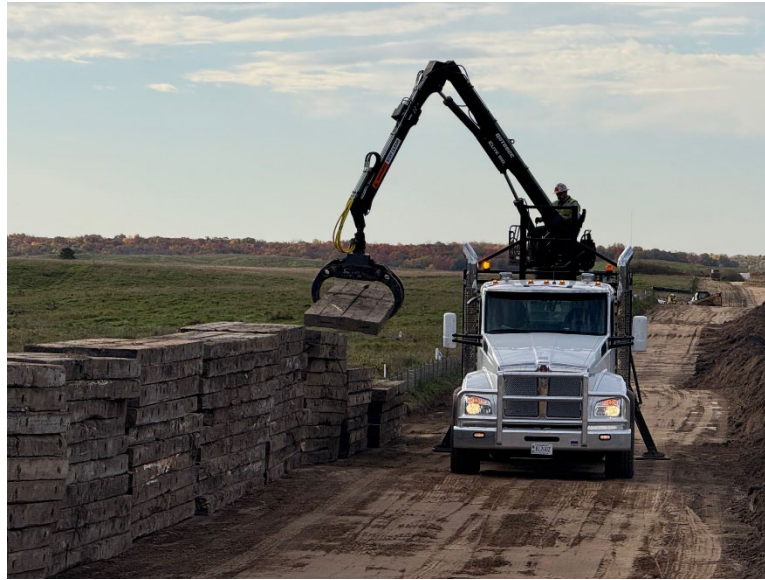
Facing south at MP 1.05, Northern Clearing Inc. continuing mat removal
