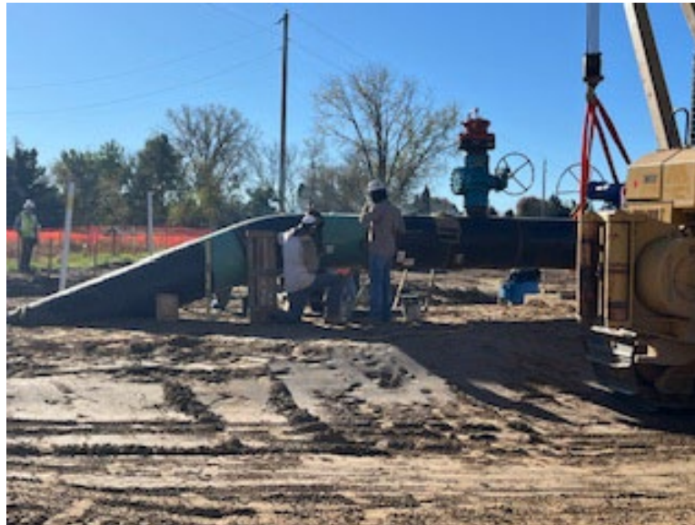
Facing east near MP 3.42, aboveground piping installed
