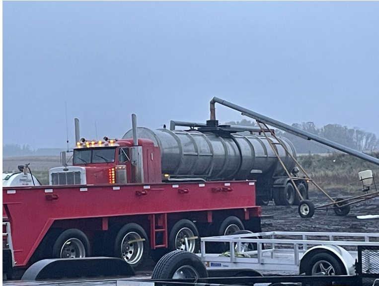
Facing northwest at milepost (MP) 34.2, K&K loading out hydrostatic test water for disposal
