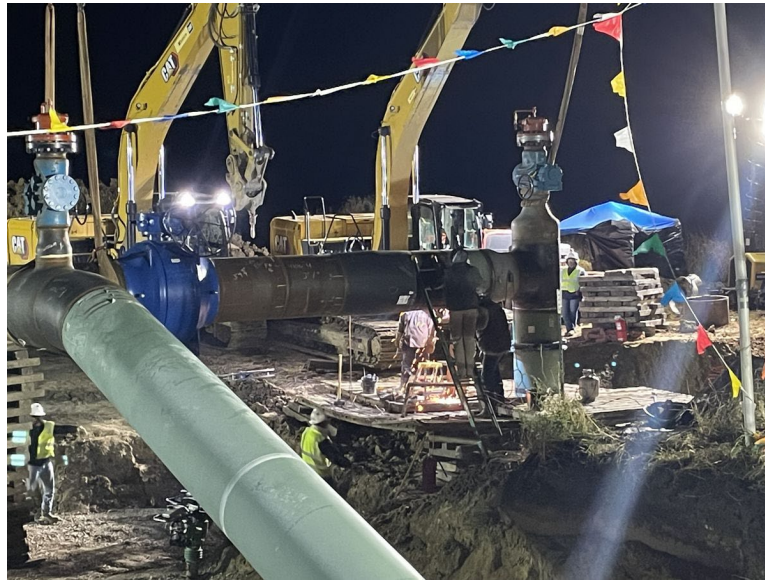
Facing northeast at MP 34.2, K&K making a tie-over weld north of 165th Street
