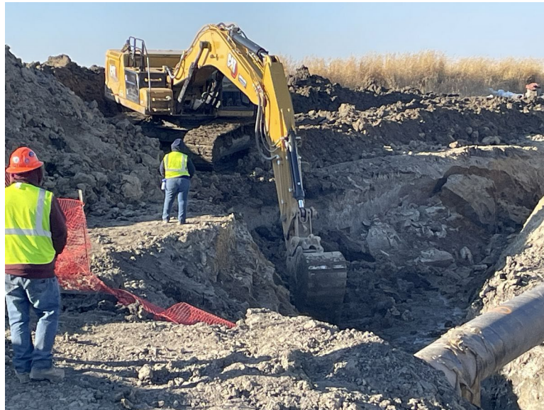
Facing northwest at MP 31.2, K&K mechanically excavating trench north of County Road 9/135th Street
