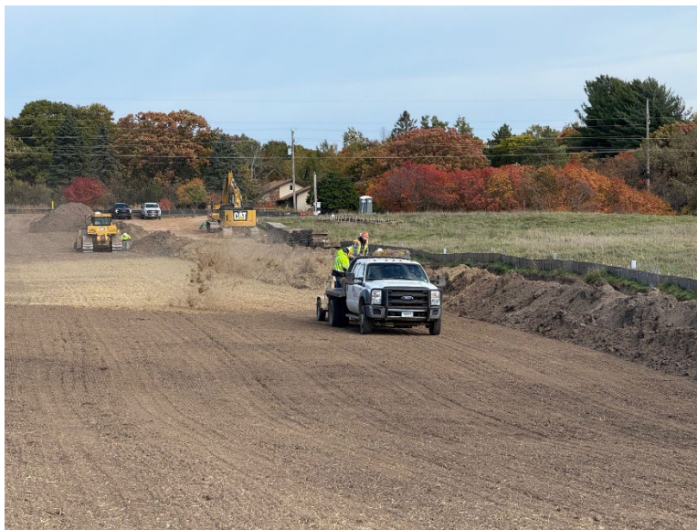
Facing north at MP 1.1, Otis seeding and mulching the ROW
